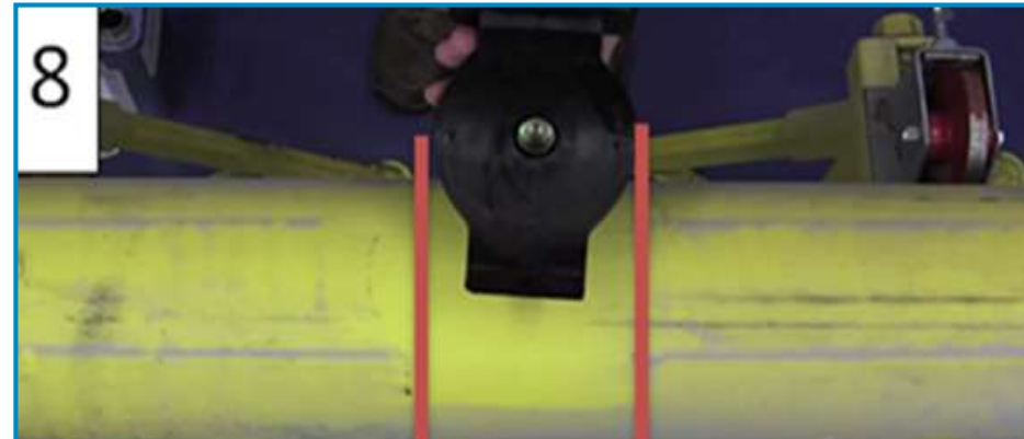
8 Presence of film of contamination on what appears to a clean pipe and fitting
