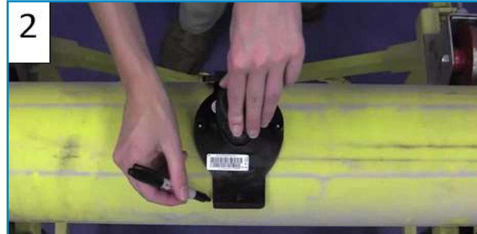
2 Establishing the fusion/scraping zone
