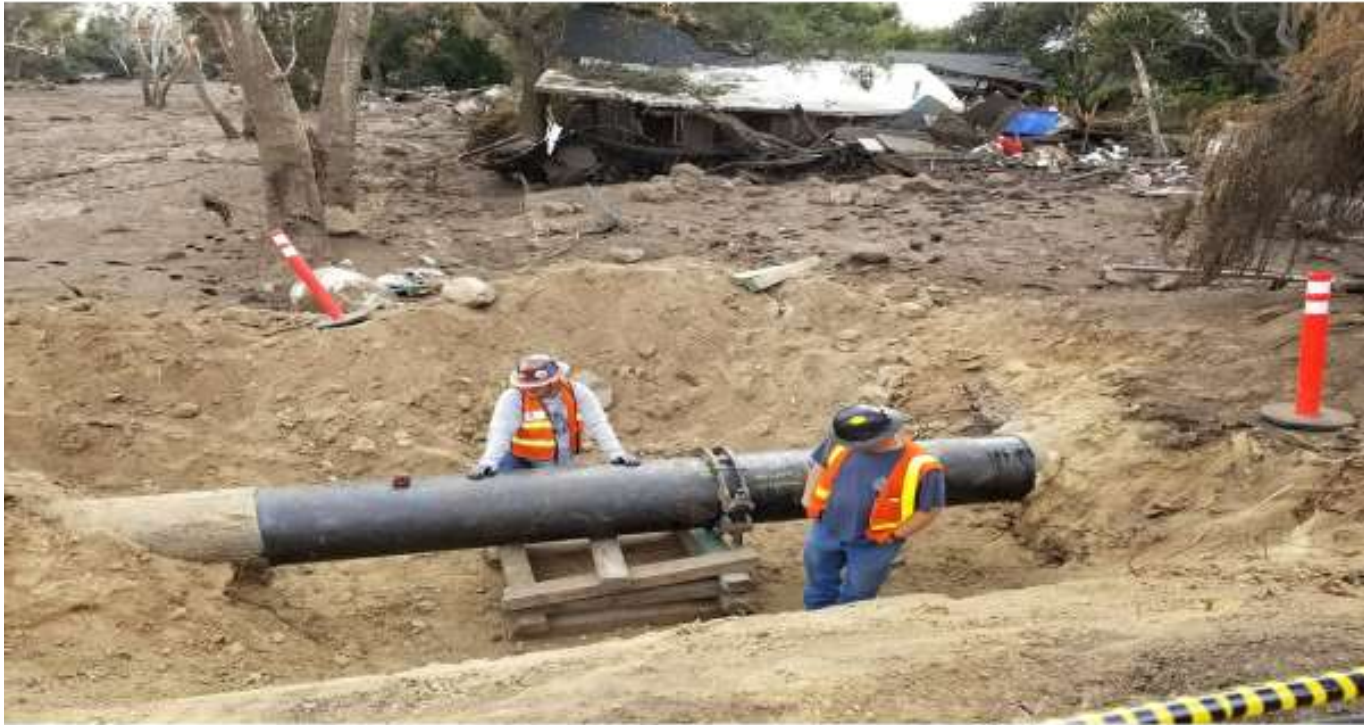
SoCalGas crew inspects gas line in area heavily impacted by mudslides.
